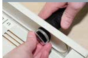
FLP conduit with sheath trimmed back
